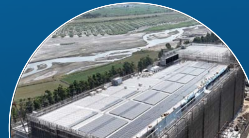
Battery Factory in Kaohsiung HeFa
